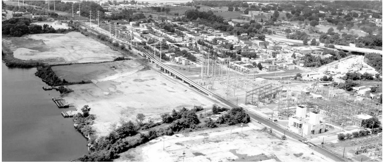
Figure 9: Existing transportation networks serve trains and automobiles but stand as barriers to neighbors attempting to access the waterfront.
