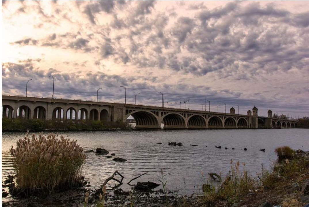
Figure 13: Hanover Street Bridge (source: Patrick Gillespie)
